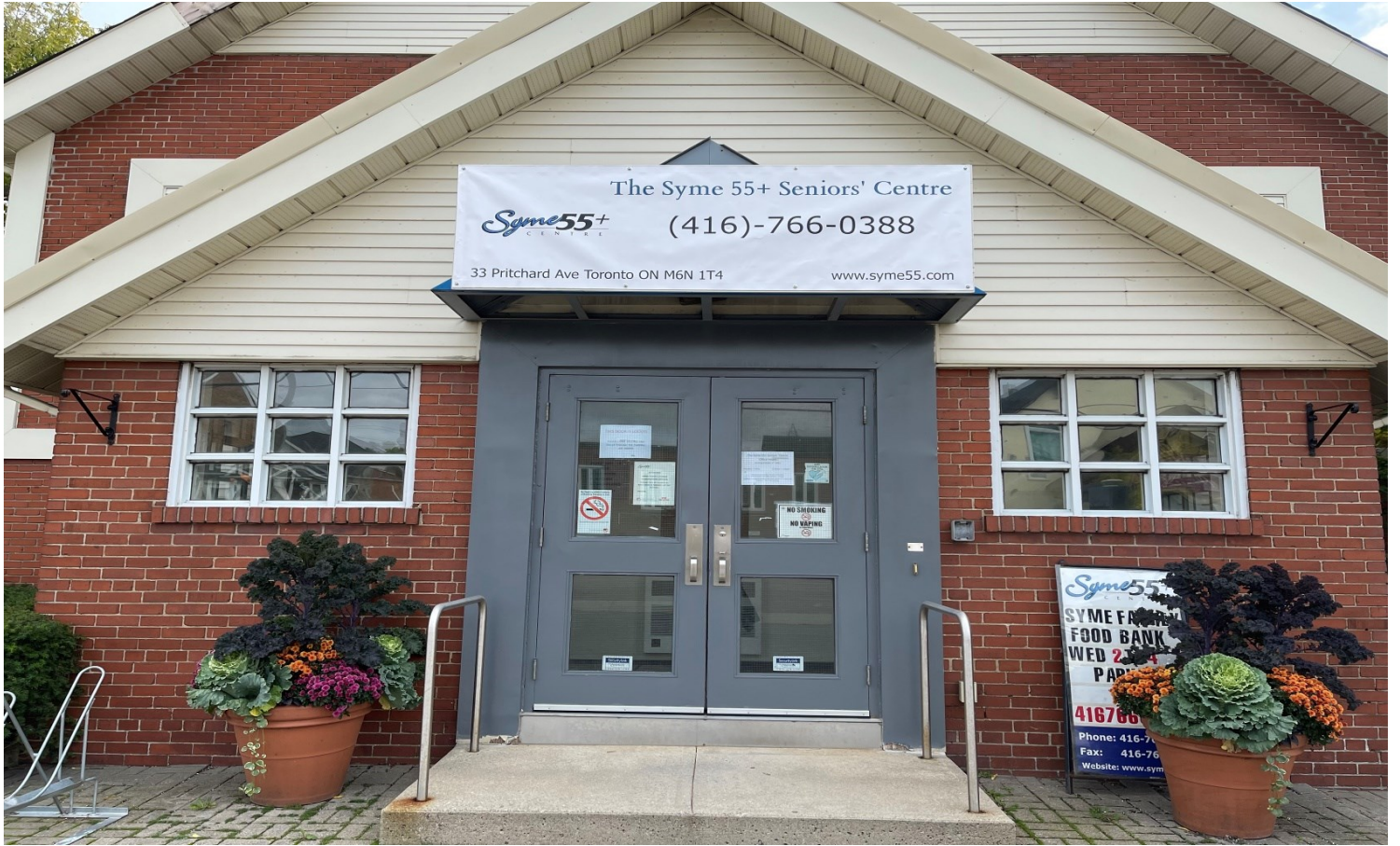
Above: facing Pritchard Ave.
